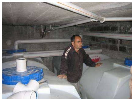
Figure 10: four urine tanks are deposit in the basement of the school (source AWHHE)
