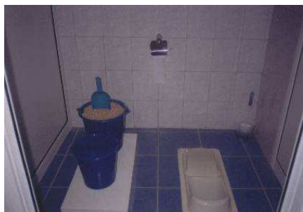
Figure 11: ecosan toilet interior (source AWHHE)
