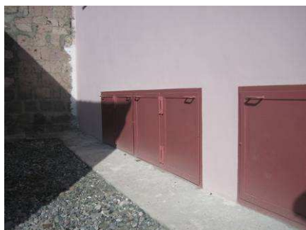
Figure 12: faeces collection chamber (source: WECF)
